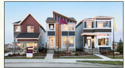
Photo courtesy of Jayman BUILT.
