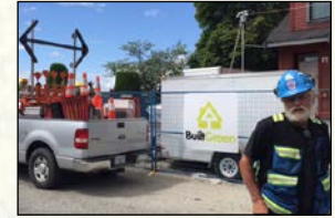
John Petzelt, Site Manager, Avalonna Homes Ltd. onsite at Avalonna Mews project.
