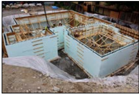
Photo courtesy of Vancouver ICF.
